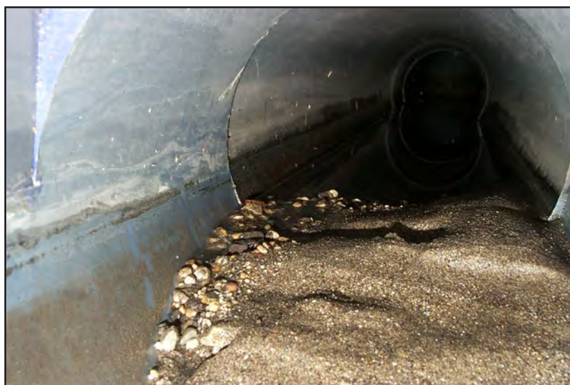
Figure 22. Cleanout of the 8-inch inlet pipe for the hydrodynamic-settling device.
